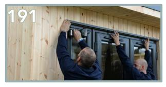
Position the top plastic 'L' strip across the door. Pre-drill the face underneath and fix first.
