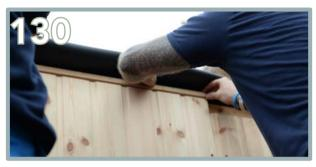
Repeat the same process for the smaller batten on top of the taller T&G side panel (BC) & (BA). Screw into place using 2 x 80mm screws. Repeat the process on the opposite side.
