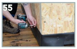
Once all of the wall panels are up, begin to secure each wall panel to the floor plate underneath. Use  $3\times35$ mm per panel externally.
