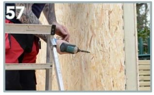
Internally position the screws each side of the adjoining split line. Use  $5 \times 35$ mm screws for each side of adjoining panels with the spline panel inside from top to bottom. Repeat this process for every adjoining panel.
