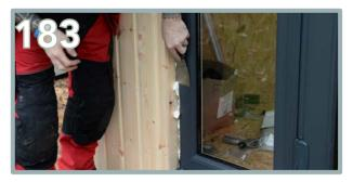
Remove all excess expanding foam around the window and door frames. Preferably it is better to wait for the expanding foam to cure before removing for easier removal.
