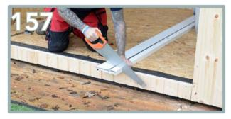
The door ledge will be oversized by 100mm. You will need to measure and cut off the excess.
