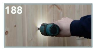
You will need to fill in the holes of each screw in the T&G panels to create a flat finish. Further countersink the screws, and enlarge the hole by 10mm.
