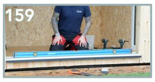
Place the ledge onto the silicone. Ensure it is level and the back edge meets the first edge of the back OSB sheet (The same positioning as the window).
