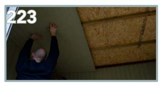
Start from the left side. Ensure the rounded edge is butted up against the side panels. You will need at least one person to hold the panel up whilst the other screws it into place.
