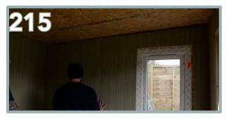
Move onto the front beaded boards. There will be two 'L' shaped pieces on either side of the door. Use 10 x 50mm screws to secure. Use 6 x 50mm screws on the top half and 4 x 50mm screws on the bottom half. Use 6 x 50mm screws for the lintel board in the middle.
