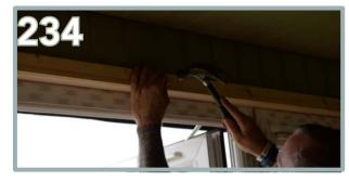
Fix into place using 6 x 30mm nails.
