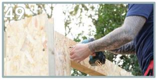
Position the screws on the wall panels OSB and screw into the window insert batten behind.
