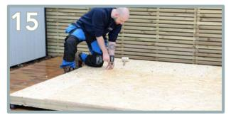
Using 35mm screws, screw 3 across the top and 5 down the sides of each OSB sheet. Screw along the edges first.
