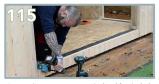
Repeat the same process as the lintel for the kick plate panel (BK) that goes underneath the door opening.
