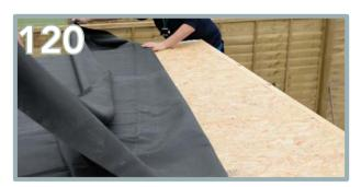
Fold the EPDM back to half way across the roof - we recommend two people for this. Be careful when moving on and around the roof to prevent any possible injuries.
