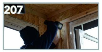
Then apply a batten in between the other two. Use 4 x 80mm screws and repeat on the opposite side of the door.
