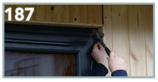
Secure into place with 5 x 30mm nails. Repeat the process for the opposite side of the door frame. Then repeat the same application around the window frame.
