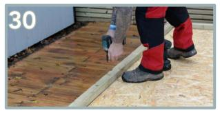
Your side floor plates (AK) will fit in between your front and back plates. Ensure 11mm from the outer edge and 11mm at each end. Once happy with the position, pre-drill and screw into place using 4 x 125mm screws.
