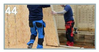
Continue on the right hand side panels as shown above (N), adding the expanding foam into the bottom grooves. Place and knock into the other side panel.
