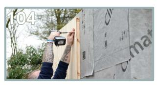
Use 6 x 80mm screws per panel. Ensure you use 3 x 80mm screws down each side of the cladded panel.
