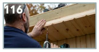
Apply the canopy panels (BJ) one at a time. Ensure they are flush to all edges. Apply 6 x 80mm screws per panel.
