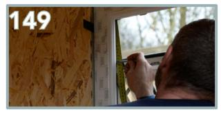
These should be drilled 150mm from the top and bottom corners and 300mm from the 150mm point at both sides. Use packers at the fixing points to avoid distortion to the frame.
