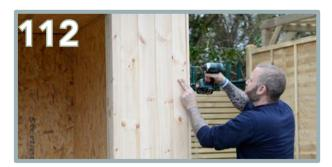
Use 3 x 80mm screws for the other edge of the side panel (BC) and screw into the front panel (AU) batten to secure together.
