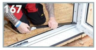
Remove the plastic strips from the bottom of the door frame. Keep hold of these pieces to re-apply afterwards.
