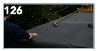
Finish with a final brush on the EPDM to produce a flat and even result.
