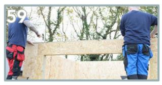
Insert the front wall plate (AL), knocking into place. Expect this to be tight fitting. Ensure it is flush to the top and ends.
