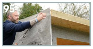
Use the excess membrane to cover the angle on the side panels.
