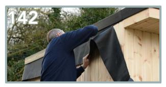
Once the plastic trims are complete around the roof, using a Stanley knife remove all of the EPDM excess. Use the plastic trims as a guide. Be careful not to cut the T&G panels behind.
