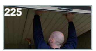
Repeat the same process. Ensure the rounded edge is butted up against the chamfered edge on the first panel.
