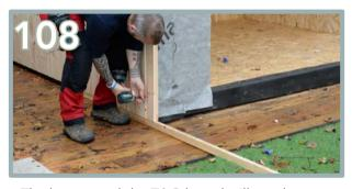
The batten and the T&G board will overhang at the front, as indicated on the layout shown above. Pre-drill ready, as these 3 x 80mm screws will go into the front panel.
