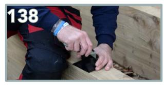
Before applying the corners onto the trims, you need to remove the plastic support. Use a Stanley knife to score an outline to weaken the support.
