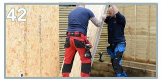
Repeat the same process for the right hand corner (G). Add foam and knock into place. Ensure the panel is flush to all edges as mentioned and shown above.
