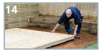
Apply OSB floor sheets (AG) on top of the SIPS panels one at a time. Ensure they are flush to all edges and screw into the corners to keep secure.
