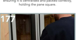
Repeat the same process for the other door and window panes, ensuring it is centralised and packed properly with the toe and heel process.
