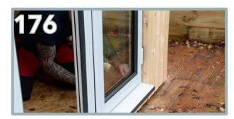
As the pane is positioned, the beading can be installed using a nylon mallet and tapped securely back into place.
