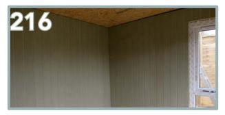
On the side panels, work from the front to the back. Ensure the window board is flush to the window edges. Then apply the next side piece. This is already trimmed for the provided space.
