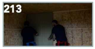
Start at the back left hand corner. Ensure the rounded edge of the panel is up against the wall. Use  $4 \times 50$ mm screws on each side and  $2 \times 50$ mm screws in the centre.
