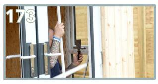
Remove the beading once again around the door, ready to insert the pane.
