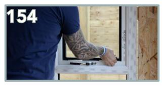
Place the top pane into position, ensuring it is centralised and packed correctly, holding the pane square.
