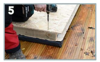
Using 125mm screws, screw through the floor panel into the floor bearer beneath. Repeat the process for the 4 other screws. Ensure each screw is countersunk.
