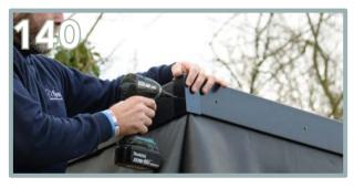
Hook and position onto the corner. Pre-drill to provide a hole for the pin.
