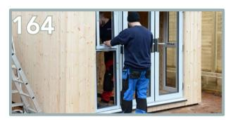
Insert the window frame into the left hand side of the double doors. The metal cap will slot into place.
