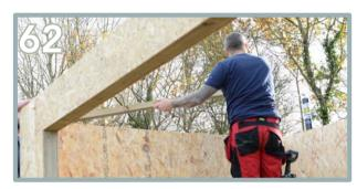
Insert the side wall plate (AK). Pre-drill and secure with 4 x 125mm screws. Repeat the process for the other side wall plate and back wall plate with expanding foam and 125mm screws.
