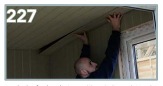
Apply the final and trimmed beaded panel. Use 8 x 50mm screws to secure.
