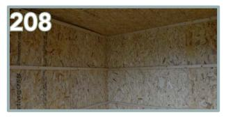
On the left hand side, apply the 45x28mm battens in between the front and back battens. These will flush end to end. Position each batten at the same height as the back.
