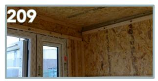
Use 5 x 80mm screws for each batten. The battens on the left hand side will not be aligned to the front batten positions.
