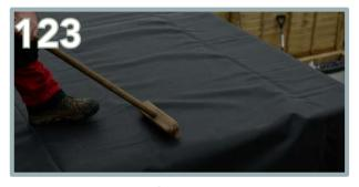
Roll the EPDM half way on to the glue. Use a brush/broom to create an even and flatter finish. You need to act quick once the glue has been applied.
