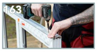
(This section is only for the 'Xtend Plus' doors and side window. This step will not apply to the standard option). Use 3 x 35mm screws to secure the metal capping.
