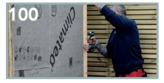
At each side, there will be a slight overhang of the T&G board. The battens edge underneath should be flush to the end. Use the 45 x 28mm batten as a guide to leave 45mm from the ground.
