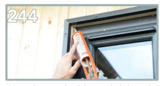
Start at the top and trail down to the ledge at the bottom. Keep the amount of silicone consistent as you trail down.
