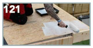
Pour the glue into a paint tray and use a roller for easier application.
