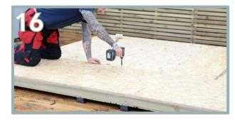
Screw the central screws into place, resulting in 3 in a row. This will result in 15 x 35mm screws per OSB sheet.
