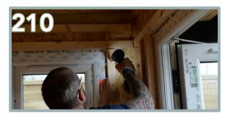
Repeat the same process for the two top battens and frame the window. Apply the 45x28x1960mm battens, one on either side using 4 x 80mm for each.
