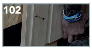
Use 6 x 80mm screws on each panel, 3 x 80mm down each side of the cladded panel, through the batten and into the wall panel behind. Leave the screws slightly out in case of adjustment.
