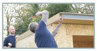
Knock further into place to allow the roof panel to be as flush as possible to the wall face.
