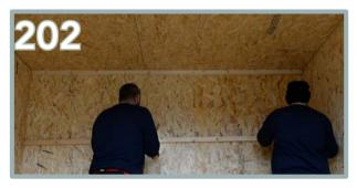
Use 5 x 80mm screws to secure equally across the batten in place.
