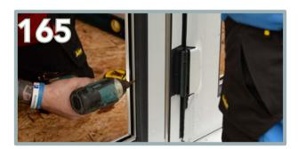
Drill 150mm from the top and bottom corners and 300mm from the 150mm points with the 112mm screws into the double doors and into the wall panel on the opposite side.
