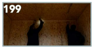
Begin at the back and position the  $45 \times 28 \text{mm}$  batten flush to the top. This will be the correct length to fit in the space end to end. Use  $5 \times 80 \text{mm}$  screws along the batten.
