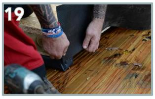
Start to unwrap the DPC roll and choose a starting point on the base's outer face. Ensure it covers half of the bearers and staple into place.
