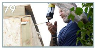
Use expanding foam in the roof panels groove across all 3 panels.
