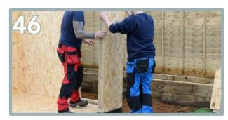
Apply the front wall panel (O) and butt up against the front side wall panel just secured. Ensure all edges are flush.
