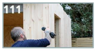
Apply the front panel (AU). Ensure it is butted up against the side panel and flush to the door section. Use 6 x 80mm screws per panel. Ensure you use 3 x 80mm screws down each side of the cladded panel.
