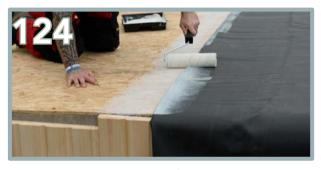
Repeat on the opposite half. Fold the EPDM back up until the point where the glue ended on the previous application.
