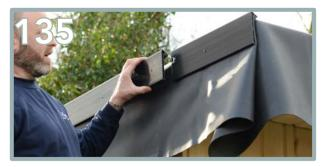
Apply the piece previously cut to size. Ensure it is flush to the front edge and butt up against the plastic trim already pinned into place.
