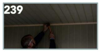
Apply the small trims at the front and back first. Ensure the trims are flush end to end and they are in contact with the roof as much as possible. Use 5 x 30mm nails.
