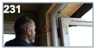
Apply the internal sides on either side of the door. Trim to fit if necessary. Use 5 x 60mm nails for each board to secure.
