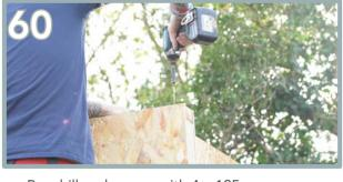
Pre-drill and secure with 4 x 125mm screws. Repeat the same process for the back wall plate (AL).
