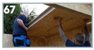
Lift up the first roof panel (V). Ensure at least 2 adults can lift up the roof panels carefully. Measure the overall width for the roof and allow 2mm each side in case of a slight oversize in roof panels.
