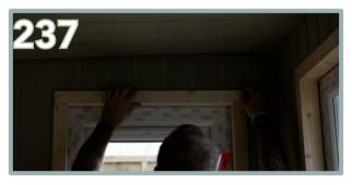
Apply the overlapping framing. Ensure flush around all edges and trim if necessary.
