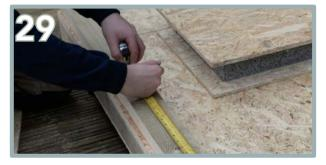
Mark and cut off the excess timber from the front floor plate. This will remove any timber from your door opening.
