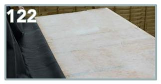
Apply glue to half of the roof and ensure to reach up to all of the edges.
