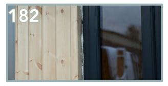
The expanding foam will be tack free in about 20 minutes. It can be cut back after twelve hours and will be fully cured in 12 -24 hours.
