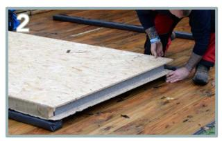
Place the first floor panel (B) on top of the two bearers and position it half way onto the second bearer. The black side covered in tar will be on top of the bearers as shown above.
