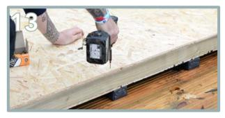
Pre-drill and use 4 x 125mm screws and ensure each screw goes into the bearer beneath. Screw 35mm screws in between the 125mm screws. Repeat process for the other floor capping.
