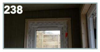
Use  $5 \times 30$ mm nails per side 45mm board. Finish with the top board using  $4 \times 30$ mm nails to secure.
