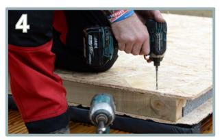
Pre-drill for every process before securing with screws. Pre-drill 5 holes along the edge of the first floor panel. Do not screw in the other side at the moment.
