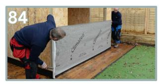
Starting with the bottom section, pull the membrane tightly and staple into place.
