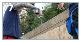
Repeat the same process as the first roof panel using  $4 \times 150$ mm screws along the edge to fully secure the roof. Then secure the second roof panels opposite corners with  $2 \times 150$ mm screws.
