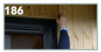
Using 6 x 30mm nails, secure the top board into the lintel. Repeat the same process for trimming the sides.
