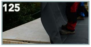
Continue with the glue application on the OSB roof surface as much as possible.
