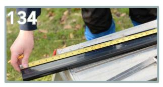
The other plastic trims will need to be measured out and cut using a hand saw to fit next to the fixed roof trim. Further detail will be shown throughout the application of the trims below.
