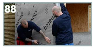
Repeat the same process for the top half of the building. Ensure the starting point is flush to the top of the back wall panels.
