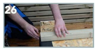
Starting with the back floor plate (AL), ensure it's flush end to end and provide 11mm spacing from the bases' back edge. Pre-drill and screw 4 x 125mm screws along the timber.
