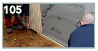
Ensure the cladded panels are 45mm off the ground. If you are using the batten as a guide, slightly lift up the secured panel to ensure it is carefully removed to prevent any damage.
