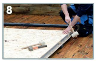
Knock on the front and back of the second panel to ensure it is flush on both edges to the first panel and floor bearers.
