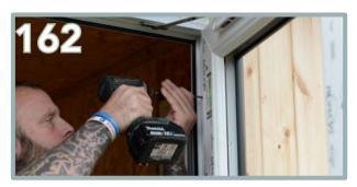
These should be drilled 150mm from the top and bottom corners and 300mm from the 150mm points with the 112mm screws.
