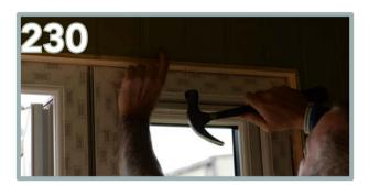
Nail into place using 6 x 30mm nails.
