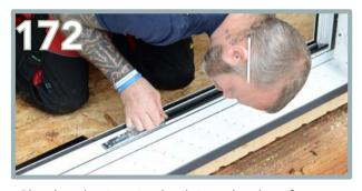
Clip the plastic strips back into the door frame to hide the screws.
