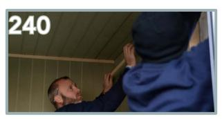
Apply the roof trims on each side, in between the front and back. Ensure these are flush end to end and follow the angle of the roof from front to back.
