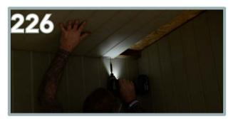
Use  $4 \times 50$ mm screws on each side and  $2 \times 50$ mm screws in the centre for both panels.
