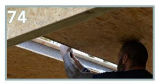
Lift up the second roof panel (U) and apply expanding foam into the inner groove as shown above.
