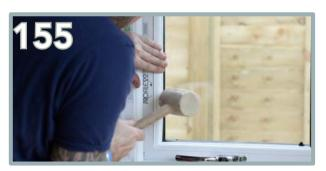
As the pane is positioned, the beading can be installed using a smaller rubber mallet and tapped securely back into place. Be careful to not aim at the glass pane.
