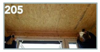
Apply one batten above the door opening, flush to the edge opening. Apply the top batten flush to the top. Use 5 x 80mm screws per batten.
