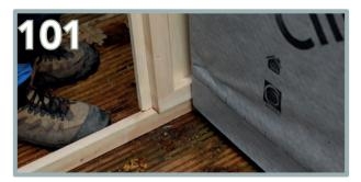
Repeat the same process for the second back panel (BM). Softly knock the second back panel into the first, so the T&G interlocks the panels together. Use a rubber mallet for a softer application.
