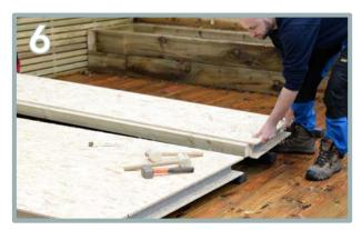
Place the second floor panel (A) onto the middle and end bearers. Ensure the panel is positioned half way on the middle bearer.
