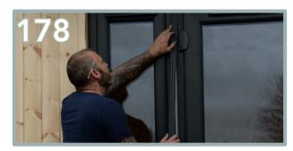
For the adjoining frames, attach the strip provided with the metal capping. This will clip into the fixed metal capping. To further secure, you can also add glue to the strip.
