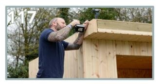
Using 2 x 80mm screws, secure the side fascia. Ensure this is flush to the top and front, whilst butting up against the T&G side panel. Repeat this process for the other side.
