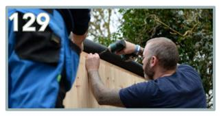
Screw into place using 2 x 80mm screws. Ensure the batten is butted up to the T&G panel and wall panel behind.
