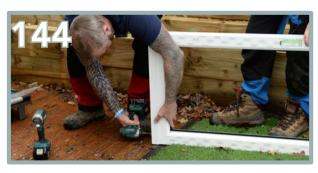
Remove any packaging from the new frame and screw the sill into the bottom of the frame. Use 2 x 50mm screws and ensure not to penetrate the inner skin of the frame.
