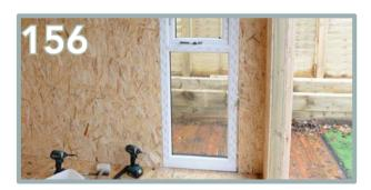
Repeat the same process for the bottom pane, ensuring it is centralised and packed properly with the toe and heel process.
