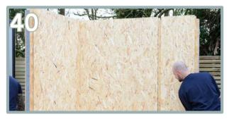
Slide the spline (Q) in the first panel (H). Please note that Xtend2.5 only has 2 x back panels.
