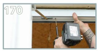
Repeat the process through the top. Drill 150mm from the both internal sides of the double doors.
