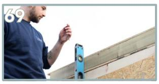
Use the spirit guide as a reference to screw through the roof panel into the side wall beneath.
