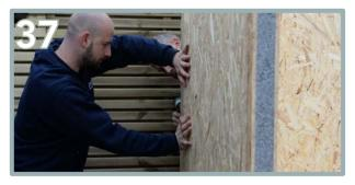
Add the expanding foam into the side groove of the Side Panel 1 (G) in the left back corner and butt it up against the first wall panel. Have one person holding onto the wall panel to prevent movement.
