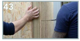
Pre-drill and screw through the back panel (H) into the side wall panel (G) using 3 x 150mm screws (top, middle and bottom).
