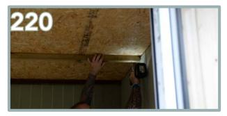
Measure and mark out equal spacing for the two central battens. Position the first batten and secure with  $5 \times 80$ mm screws.
