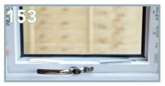
Apply packers with the adhesive silicone. The glass should be packed at diagonally opposing corners to hold the casement square, using the toe and heel process.
