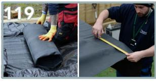
Unwrap the EPDM out onto the floor first, then measure out on the roof to ensure an equal overhang around all edges.
