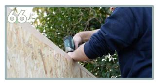
Use 2 x 35mm screws to secure the component within the thinner section. Repeat this process on the opposite side.
