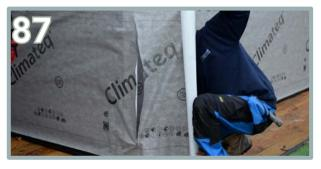
Once the starting point has been overlapped, cut off the excess and staple the end of the material into place.
