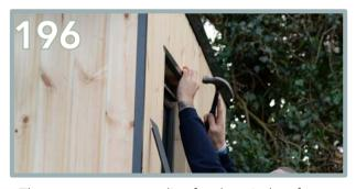
The same process applies for the window frame. Pre-drill and use 2 x pins on the front edge and 3 x pins underneath.
