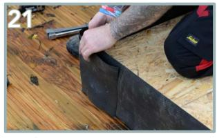
Once fully wrapped around the base, overlap the starting point and staple into place.
