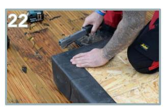
Using a Stanley knife, cut the DPC at the corner to create 2 pieces to easily fold onto the OSB sheets and staple into place.
