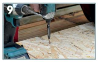
Using 4 x 35mm screws, pre-drill and screw where the adjoining panels intersect. This will secure the floor panels together.
