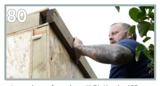
Insert the roof panel cap (AQ). Use  $4\times125$ mm screws through the panel cap and into the wall panel. Use  $3\times35$ mm screws, in between the 125mm screws to fully secure.
