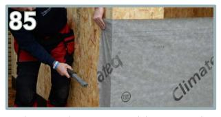
Then warp the excess around the corner and staple the starting point into place.
