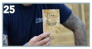
As part of your assembly pack, you will have been provided with an off cut of OSB to use as an 11mm guide when positioning the floor plates.
