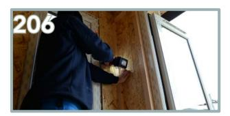
Using the 45x28x1960mm battens, apply one on each side of the door opening with  $4 \times 80$ mm screws. Then apply another two, with one in each corner, with  $4 \times 80$ mm screws.
