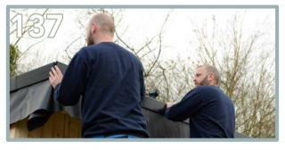
Measure and cut the plastic trims into 2 equal pieces. Ensure each end meets the side trims. Pin these into place. Add the clip in the centre of the adjoining trims.
