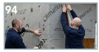
Staple into place and remove the excess from the door section.
