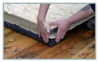
Ensure the panel is flush around the edges to the first bearer. Ensure the floor panels on the bearers are level using a spirit level as a guide.
