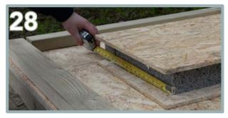
Pre-drill and use 4 x 125mm screws for the front floor plate (AL) Apply 2 x 125mm screws per end. Measure out your front panel (O) and ensure your front panel is placed flush to the edge.
