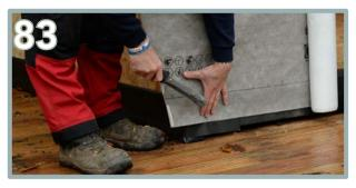
Begin to unwrap the breathable membrane. Position the membrane 45mm from the ground.
