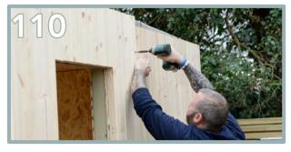
Ensure the opening of the cladding is flush around all edges to the window opening provided (BC). If not aligned properly, this will cause issues during the window installation.
