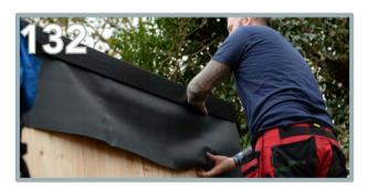
Slot the plastic trim on the top edge, flush to the back.
