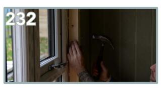
Apply the 45mm boards on top of beaded panel. Ensure this is flush to the inner framing. Use 5 x 30mm nails to secure. Repeat this process on the opposite side.
