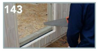
Remove the timber excess from the window section before inserting the window frame. Take out any screws in this section and cut with a saw, using the inner edge as a guide.
