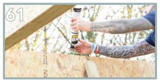
Apply expanding foam to the side panels groove.
