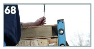
Position the back of the roof panel. Using the spirit level as a guide, the top OSB sheet on the roof panel needs to be flush to the back edge. Use 4 x 150mm screws along the edge.
