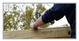
Use 4 x 80mm screws into the panel cap. Use 3 x 35mm screws, in between the 80mm screws to fully secure.
