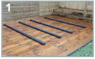
Lay the bearers down and spread them out roughly ready to position the floor panels on top.
