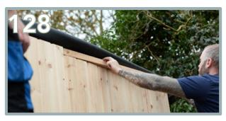
Before adding the plastic roof trims on the sides, the angled roof battens need to be applied to the gaps above the T&G panels. Fold the edge of the EPDM and slot in the batten onto the T&G side panel (BB).
