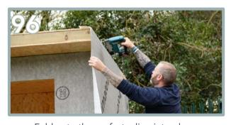
Fold onto the roof, stapling into place.
