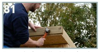
Use expanding foam and knock the roof panel cap (AQ) into place. Repeat the same process. Ensure they are flush to all edges.
