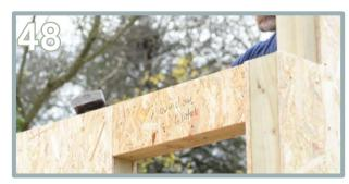
Knock the window insert (AA) into the section provided. Ensure the top is flush.
