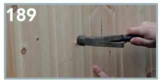
In your fixing box, there will be wood plugs. Insert one at a time, snap off and hammer further into the hole.
