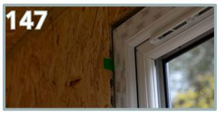
Insert packers underneath to level it and maintain the 5mm expansion gap. Ensure the back of the frame is in line with the OSB sheet inner face as shown above.
