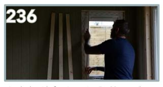
Apply the side framing, using 5 x 30mm nails per board.
