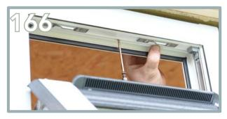
Further secure the window with  $1 \times 112$ mm screw into the top and  $1 \times 112$ mm into the bottom.
