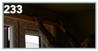
The top frame will sit on top of the side boards. Ensure both ends are flush to the side framing edge. Trim if necessary.
