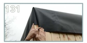
Fold the EPDM in a tucked position as shown above.
