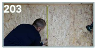
Repeat the same process to measure and mark out the position for the final back batten.
