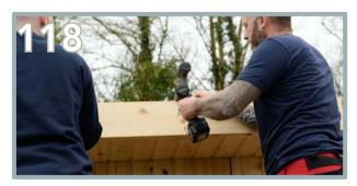
Position the front fascia. Ensure it is flush to the top and to the side fascia's outer face. Use 3 x 80mm screws centrally across the fascia. Repeat this process for the other front fascia.
