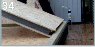
Begin the build at the left back corner, starting with Side Panel 2 (H). Insert the expanding foam provided into the bottom groove.
