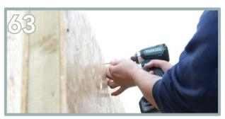
Further secure each all of the wall plates with 3 x 35mm screws externally and internally, through the OSB into the plate, in between the 125mm screws.
