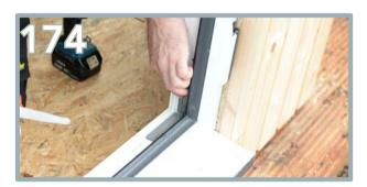
The glass should be packed using the toe and heel process. Toe and heeling works by supporting the double glazed unit with the packers.
