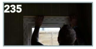
Repeat the same process for the window framing. Use  $4 \times 30$ mm nails to secure.
