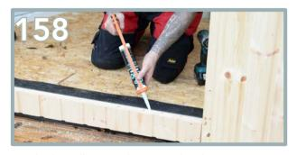
Apply the adhesive silicone in the door section. Be sure to seal the ends of sill and frame assembly to prevent moisture from tracking along the sill and into the wood work.
