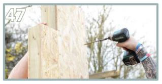
Position the screw roughly 45mm from the outer edge. Pre-drill and screw through the front into the side wall panel using 3 x 150mm screws (top, middle and bottom).
