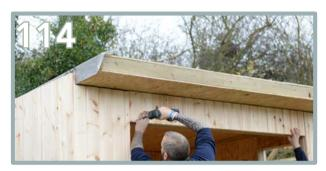
Apply the lintel panel (BL). This will fit in between the front panels. Use 6 x 80mm screws. Make sure to drill through the battens beneath.
