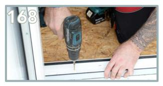
Drill 150mm from the both internal sides of the double doors. Use 112mm screws to screw into place at each side into the bottom of the frame as shown above.
