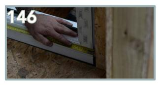
Apply adhesive silicone on to the base and carefully position the new frame into the aperture.
