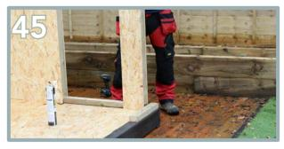
Apply the side wall panel (N1) as shown above, leaving the provided space for the window insert.
