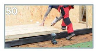
Apply the last left hand side panel (J). Apply expanding foam into the bottom groove.
