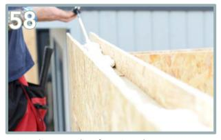
Use the expanding foam into the top groove, ready for the wall plates. Start at the front.
