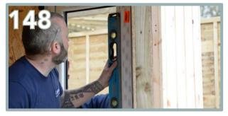
Check that frame is both level and plumb, then drill fixing holes into the frame sides. Pre-drill with a 6.5mm drill bit.
