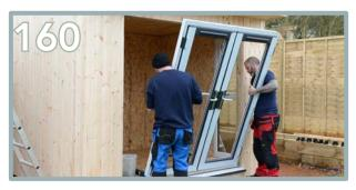
Lift and angle the frame and sit into the ledge. Butt up against the wall panel.
