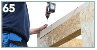
Use 2 x 125mm screws to secure the component within the thicker section.
