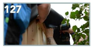
Underneath the EPDM, you will need to secure the back roof battens to the back T&G Panels (BM & BN). Ensure the battens edge is flush to the top of the T&G Panel. Secure with 3 x 80mm screws per batten.
