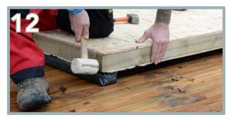
Insert and knock the floor capping (AL) into place using a rubber mallet. Ensure it is flush to all edges.
