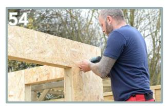
Position the screws on the Lintels OSB and screw into the wall batten behind. Secure into place using 4 x 35mm screws internally and externally, 2 x 35mm screws each side of the lintel insert.
