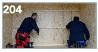
Using  $5 \times 80$ mm screws to secure in place.
