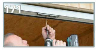
Repeat the same process centrally. Screw 1 x 112mm screw in the centre.
