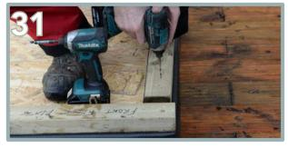
Repeat the process on the other side floor plate (AK) and screw into place.
