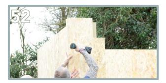
Apply the other front wall panel (O). Pre-drill and screw through the front into the side wall panel using 3 x 150mm screws (top, middle and bottom).
