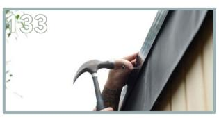
Use the pins provided with the plastic trims. Pin into the batten behind to secure in place.
