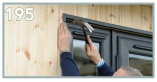
Use  $5 \times pins$  on the front down the side strip. Repeat the same process for the opposite side.
