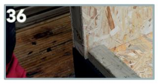
In the left hand corner, the wall panel will be flush to the edge and the floor plate as shown above.
