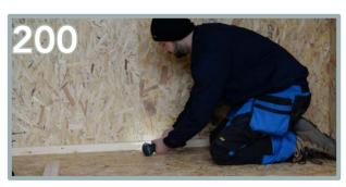
Repeat the process with the batten being flush to the bottom and end to end. Use 5 x 80mm screws along the batten at equal spaces.
