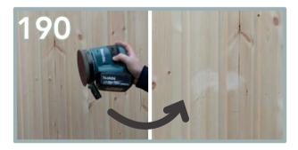
Finish with slightly cutting down and/or just sanding off any excess showing to produce a seamless finish. Repeat this process for every screw hole on the T&G panels.
