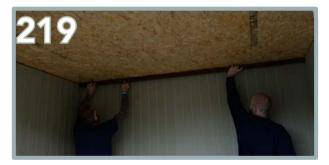
Apply the 45x45mm roof battens. Start at the back. Ensure it is flush end to end and against the back beaded panels. Secure with 5 x 80mm screws. Repeat the same process as the front.
