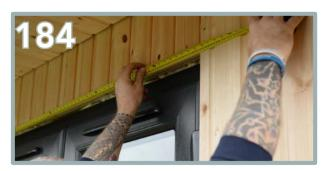
If any of the boards are slightly oversized, you will need to measure out your required length. Start with the top board.
