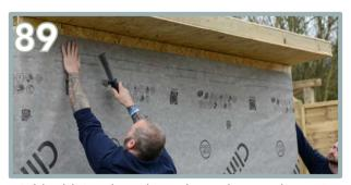
Add additional staples to keep the membrane in place. Be careful not to staple into the door and window gaps.
