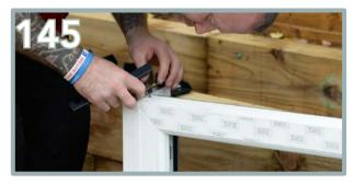
Be sure to seal the ends of sill with the caps provided to prevent moisture from tracking along into the wood work.
