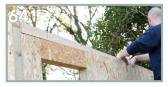
Position the firring (AB) and butt up against the front wall panel.
