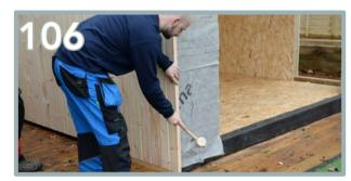
Apply the next side panel (BA). Softly knock the second side panel into the first, so the T&G interlocks the panels together. Use a rubber mallet for a softer application.
