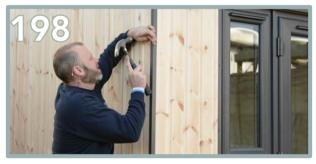
Add strips to each of the corners. The two on the back corners will be shorter. Trim to length if necessary and use 4 x pins.
