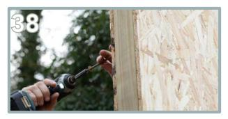
Pre-drill and using the star drill bit provided in your fixing box, screw through the back into the side wall panel using 3 x 150mm screws (top, middle and bottom).
