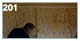
Measure and mark out even spaces to position the two middle battens.
