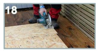
Some pieces may be oversized. If this is the case, saw the excess off after the piece is screwed into place, to create a flush finish.
