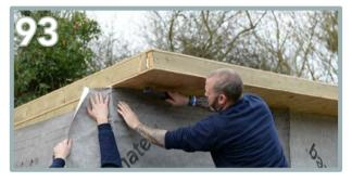
Using the excess membrane, cover the front flush up to the roof.
