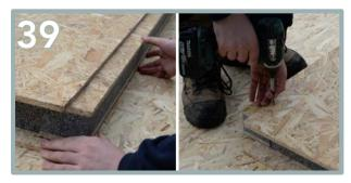
There will be smaller Spline panels (Q) that will be in between the grooves of some panels. Add expanding foam into each groove of the spline panel and apply them accordingly to the wall panel layout. Secure with 5 x 35mm screws.
