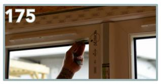
Apply silicone and stick the packers at diagonal opposing corners. Place the pane into position, ensuring it is centralised and packed correctly, holding the pane square.
