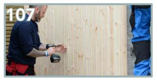
Using 3  $\times$  80mm screws, screw the one side into place.
