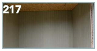
Use 10 x 50mm screws for the window panel and the trimmed side panel. Repeat the same process on the opposite side. Both of these will be the same sizes to fit into place.
