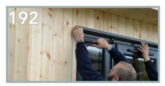
Using the pins provided with the trims, apply 2 in each corner and 1 x pin in the middle.
