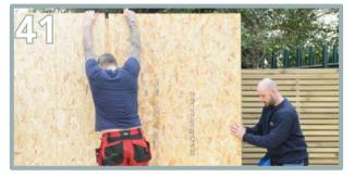
Add expanding foam into the inner side groove and into the bottom groove of the second back panel (H) and knock into place to complete the back wall.
