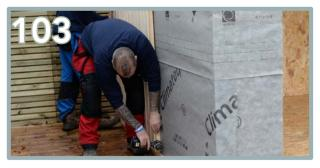
Continue onto the side panels (BB). Knock the first panel in place and ensure it is butted up against the back panel overhang.
