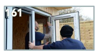
Check that frame is both level and plumb, then drill fixing holes into the frame side.
