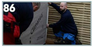
Continue unwrapping the membrane, pulling tightly and stapling into place.
