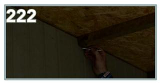
Mark out a guide line underneath all the battens at both ends. This will help when applying the roof panels and ensuring that you drill into the battens behind.
