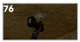
Pre-drill and screw 5 x 35mm screws, where the adjoining panels intersect.
