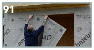
Using a Stanley knife, remove the excess from the door section, using the walls as a guide to ensure it is cut straight.
